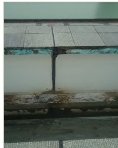
Figure 8: No leakage point for 24 hours at full water level.
