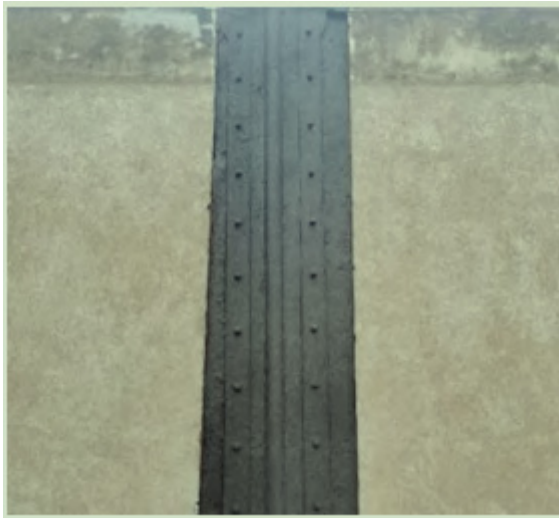
Figure 9: Waterproof paint coating
