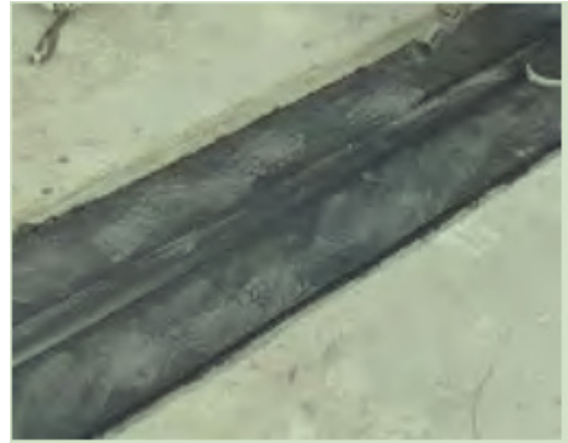
Figure 6: EPDM Ω-shaped waterstop
