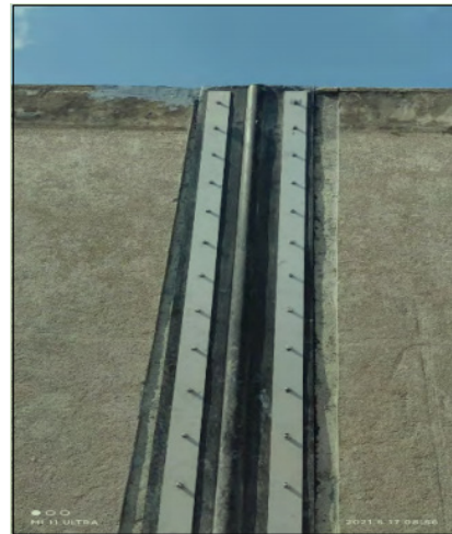
Figure 7: The construction of stainless steel bead is completed.
